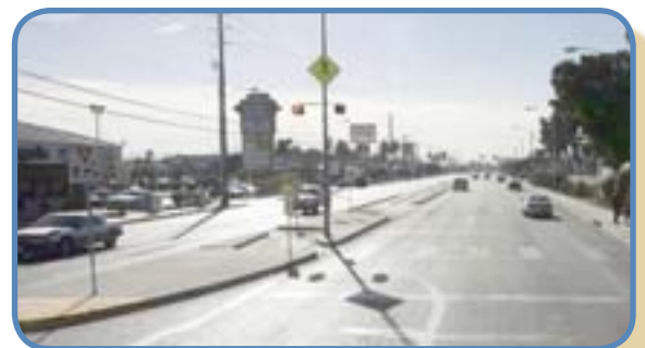
medians, signs, and signals
